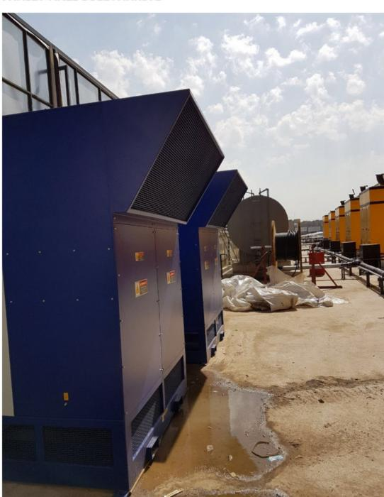
Familly Mall have 2,5MW (10x2500Kva) powered diesel generators, however generators on site was working with %30 capacity. While using 2x500KW loadbanks they save the gensets and increased the power usage.
